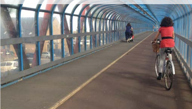
Figure 10.50: Covered pedestrian/cycle bridge across railway tracks, Cambridge
