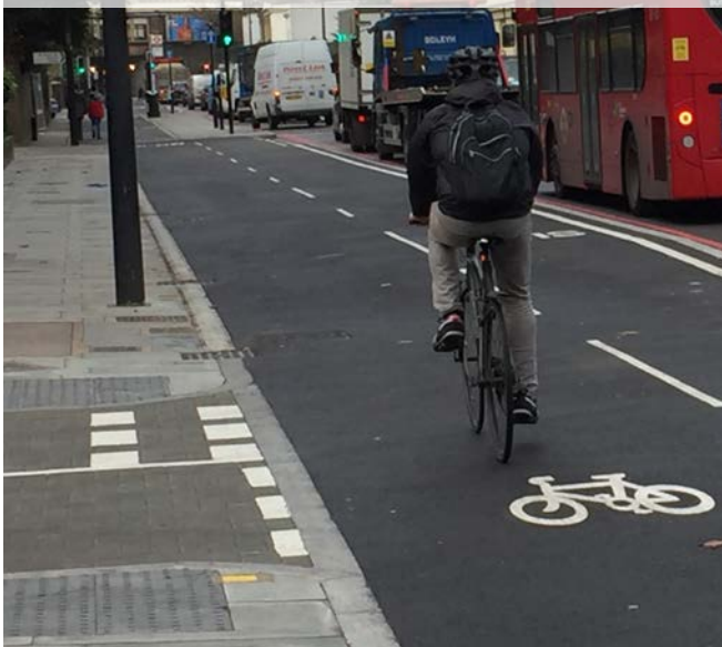
Figure 7.10: Tight kerb radii at residential side street
