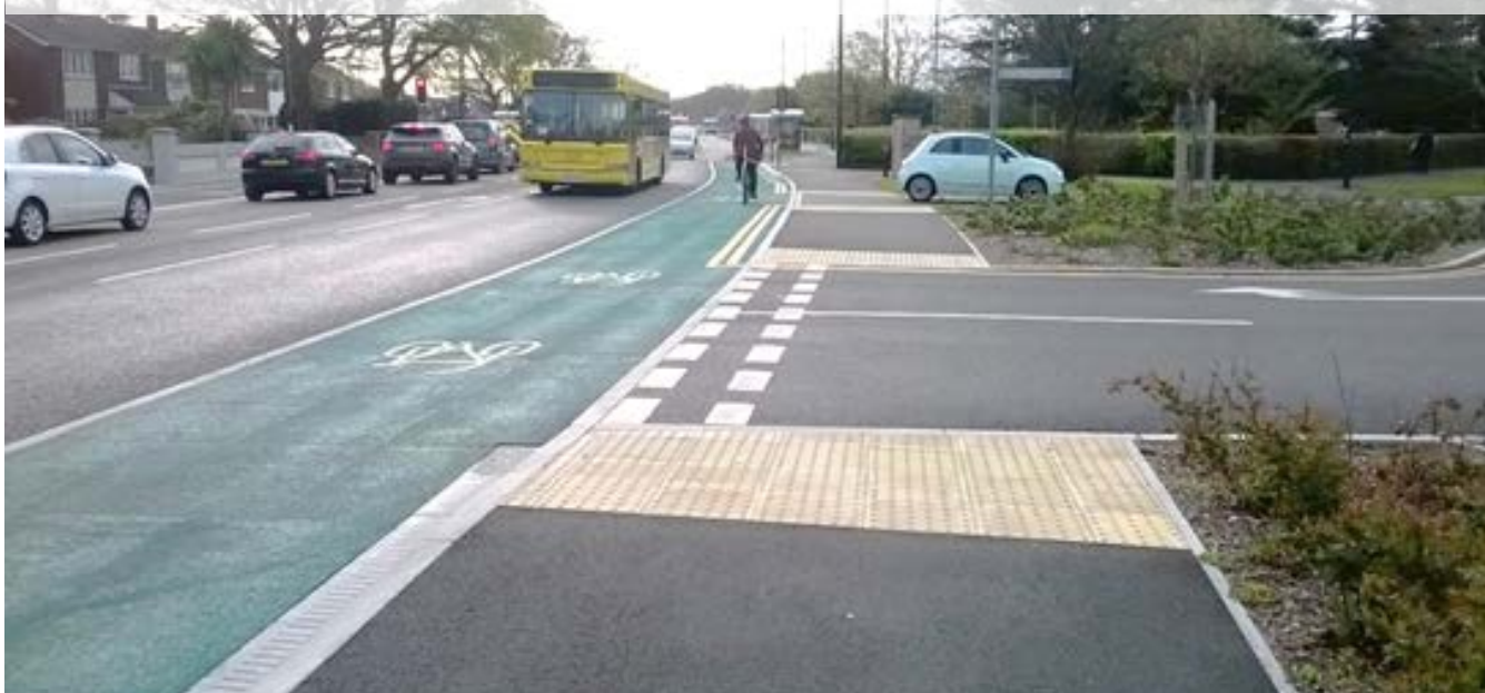
Figure 10.17: No setback crossing with design priority,– Bournemouth
