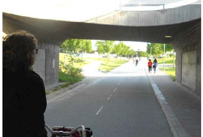
Figure: 10.52 Underbridge (cycle and pedestrian-only) with divided carriageway above to create opening – Lund, Sweden
