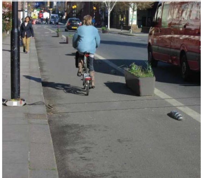
Figure 6.16: Light segregation using planters and low level features, Camden
