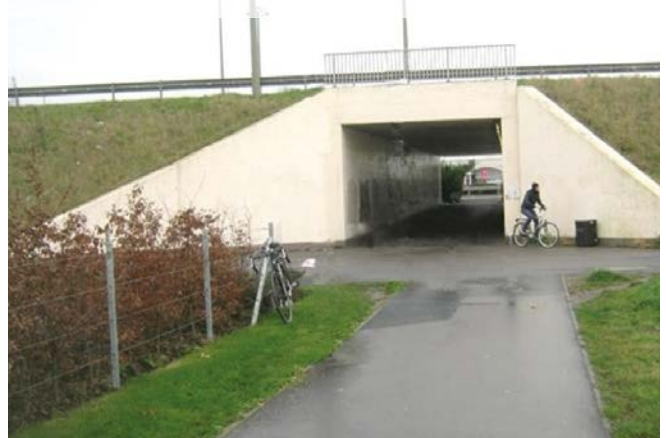
Figure 10.51 Underbridge near Cowley on Oxford Bypass with at-grade approach, wing walls and clear sightlines
