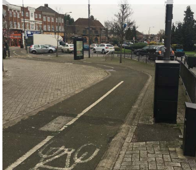
Figure 10.36: Footway-level cycle track around large roundabout, Harrow
