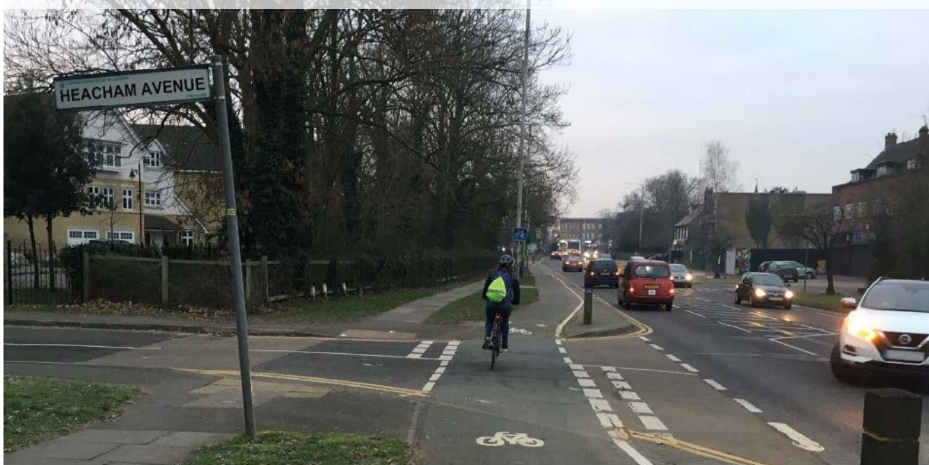
Figure 10.16: Partial set back, marked priority crossing, Hillingdon
